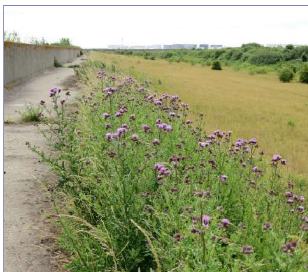
Sea wall at Coryton, Essex © Steven Falk
