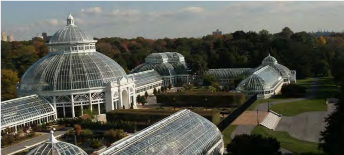
The Dome's compression ring needs replacement.
