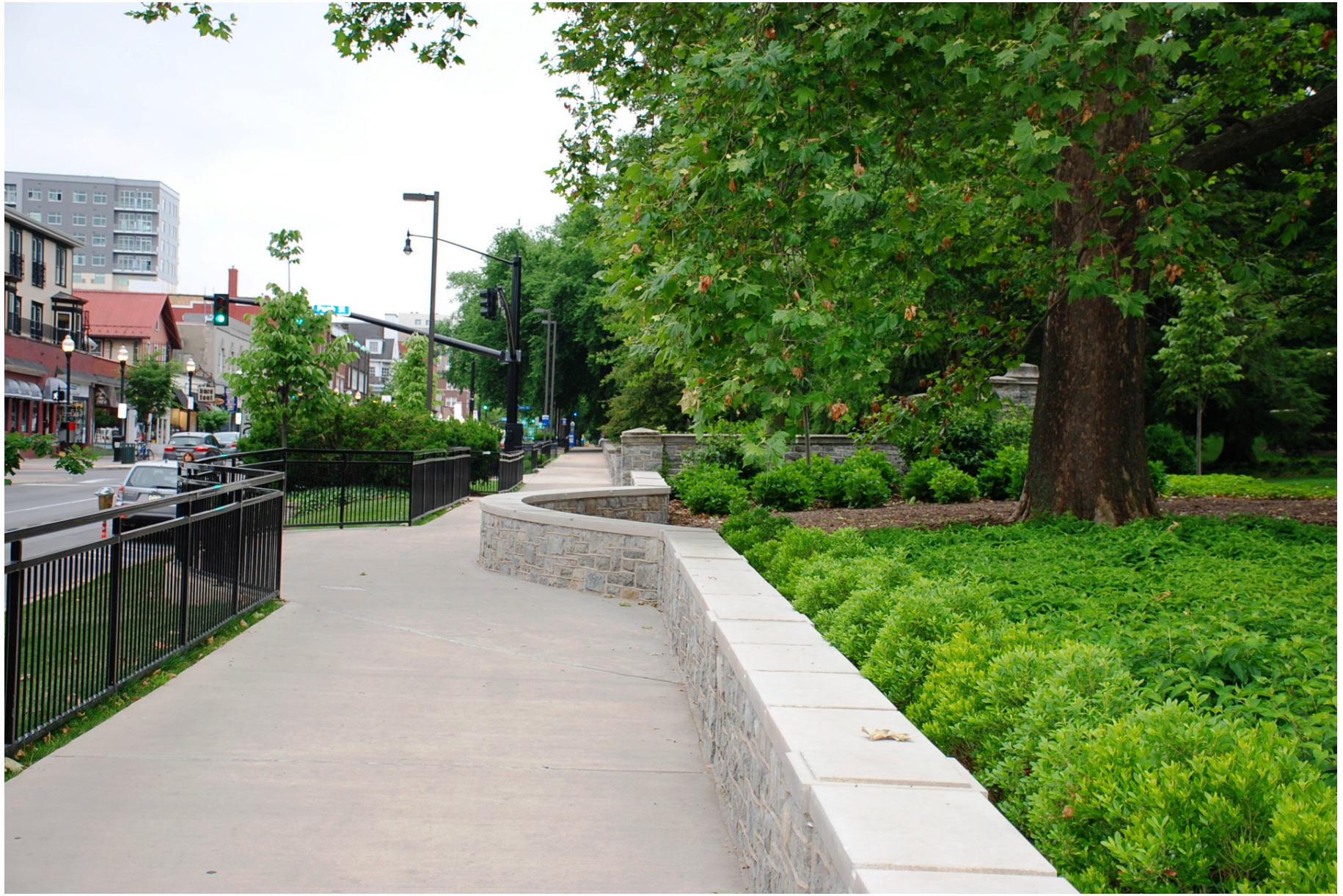
Tree Protection During Construction
