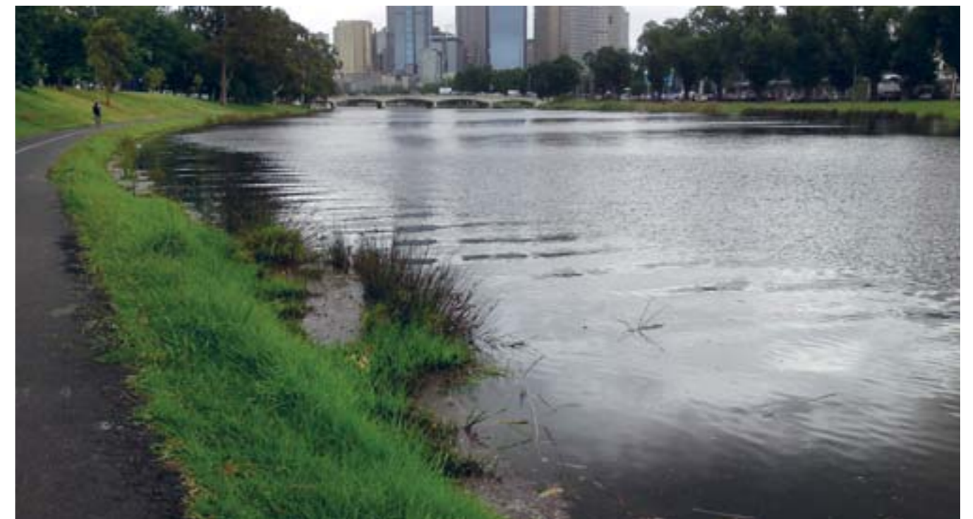
Figure 16 Very high water level in the Yarra River on 9 December 2012, when brackish water flowed back through the outlet into the Ornamental Lake
