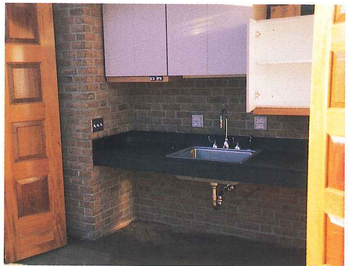
An accessible sink and adjustable cabinets are just two of the design features of the outdoor work station.
